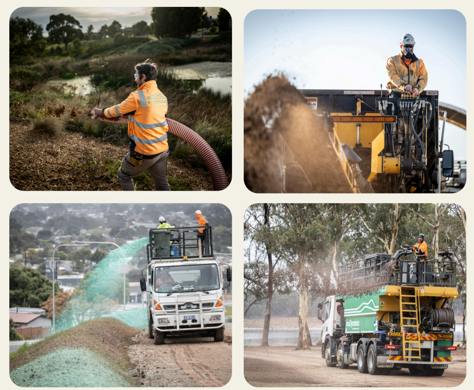
Blowing | Slinging | Hydroseeding/Hydromulching
